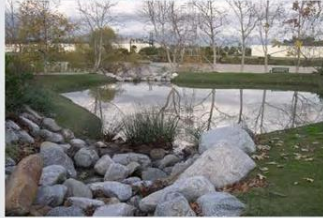
Biodetention with Underdrains
