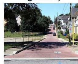
Permeable Pavement (NBS / Not Vegetated)
