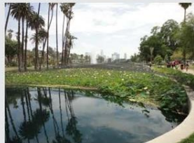
Wet and Dry Detention Basins
